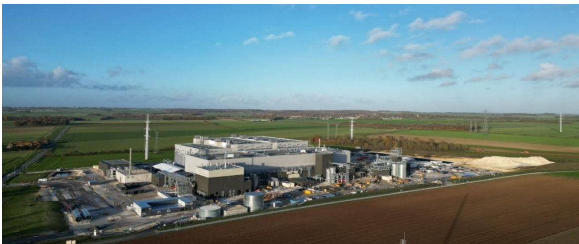
Figure 9 FARMYNG flagship plant (Poulainville, France).
